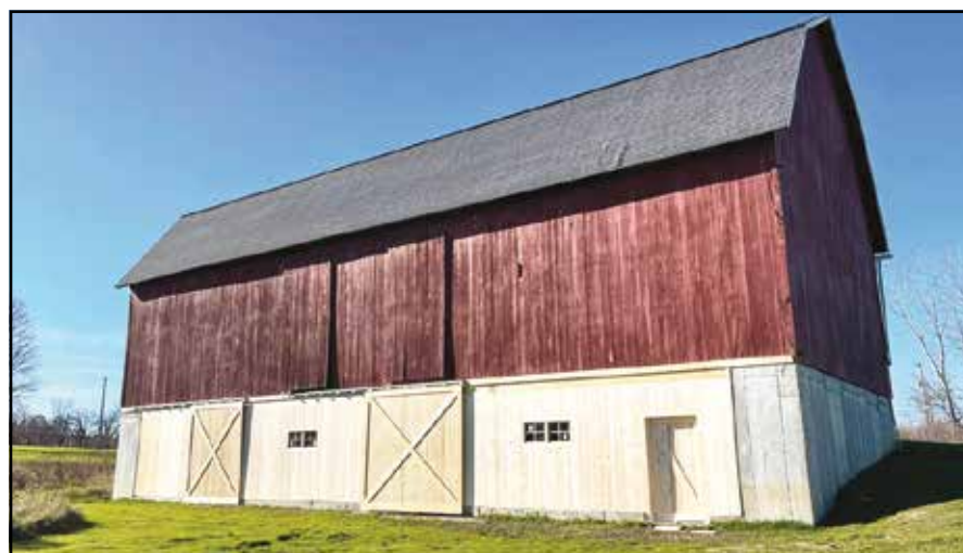
Holly Township awarded a contract to Hillman Roofing, LLC to reroof the historic Holly Heritage Farmstead barn.
