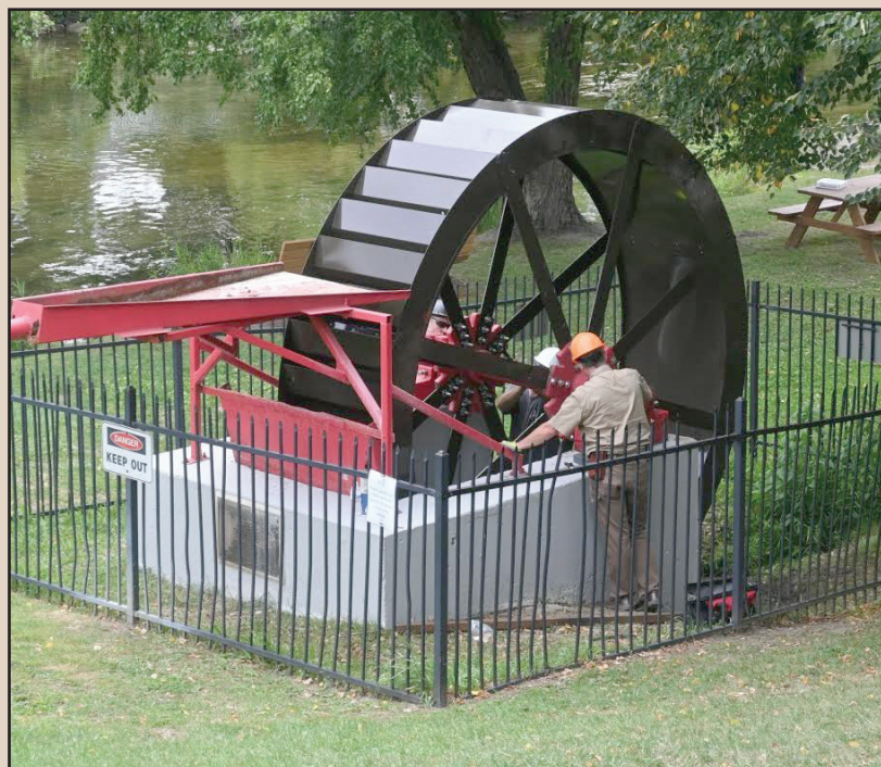
On Monday, Aug. 29, Waterwheel Manufacturing installed the restored water wheel in downtown Linden at the Kimble-Sharp Park. Submitted photo
