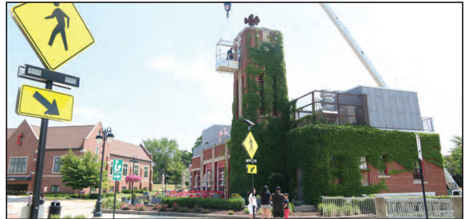
Repairs to the clock on the clock tower on the Fenton Fire Hall restaurant, and former Fenton fire station, are nearly complete. Photo: Hannah Ball
