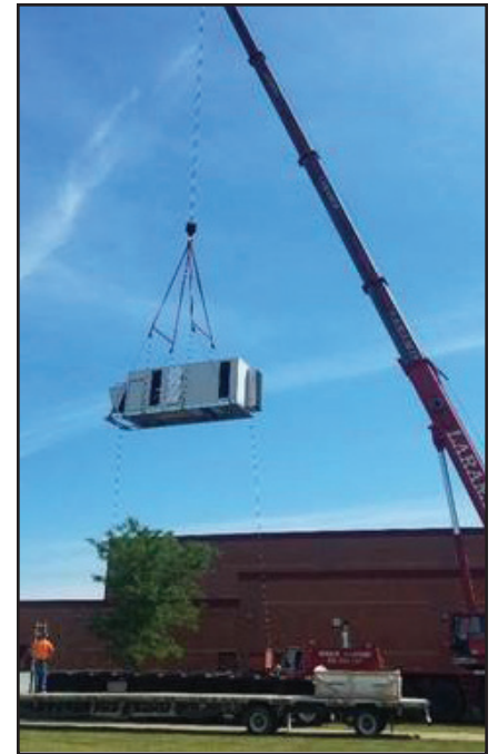
A new dehumidification unit is lifted into place for the Holly High School pool. Submitted photo
