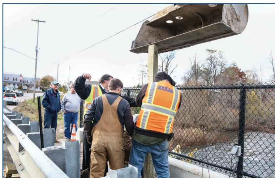
Workers with the Genesee County Road Commission and Zito Construction manage to close the broken gate in the Argentine Township dam. The structure manages water for Bennett and Lobdell lakes, which then flows to Byron. Photo: Hannah Ball
