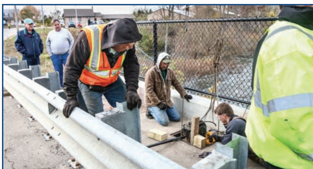
An employee with Zito Construction saws out the broken operator shaft from the Argentine Township dam on Tuesday, Nov. 5. Photo: Hannah Ball
