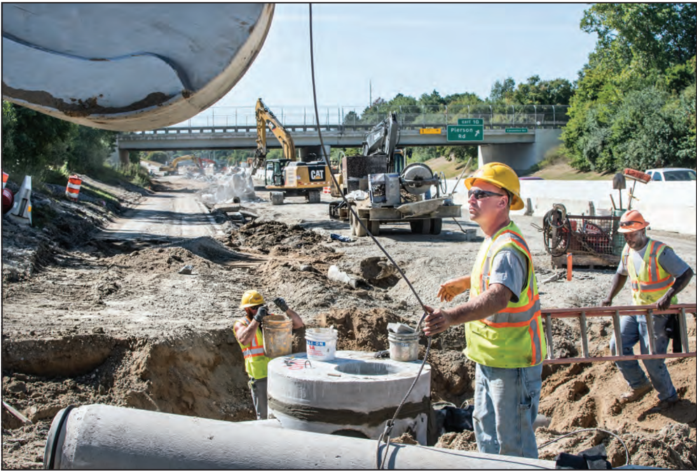
Workers with Dan's Excavating, Inc. install storm drains under northbound I-475 in Flint on Thursday, Aug. 29. This section is part of the 50-year pavement design. Photo: Tim Jagielo
