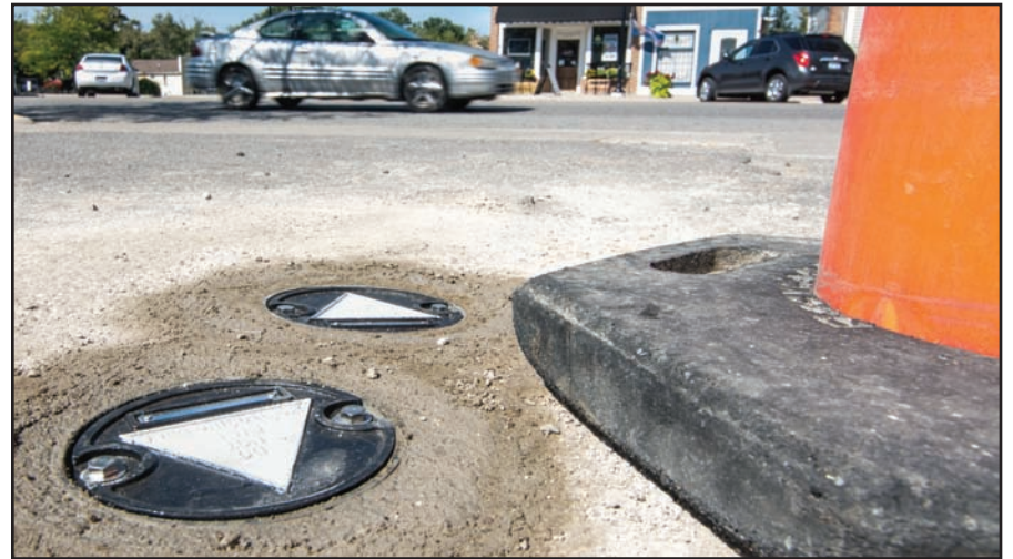
The Department of Environmental Quality installed monitoring wells in downtown Linden in September 2015 after the discovery of an underground gasoline leak.
