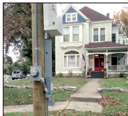
This is a sample of a small cell tower located in a town's right of way. Photo: www.INSIDERLOUISEVILLE.COM
