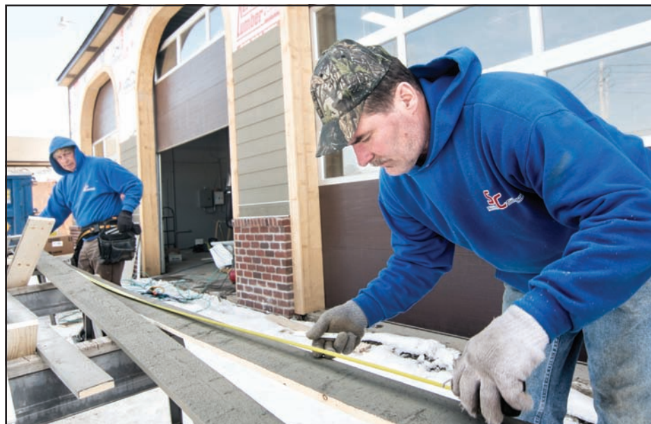
Carpenters Frank Satkowiak (right) and Mike Grajcar measure and cut cement siding for the new Holly Fire Department headquarters Friday, March 8. The building will be occupied within a few weeks. Photo: Tim Jagielo
