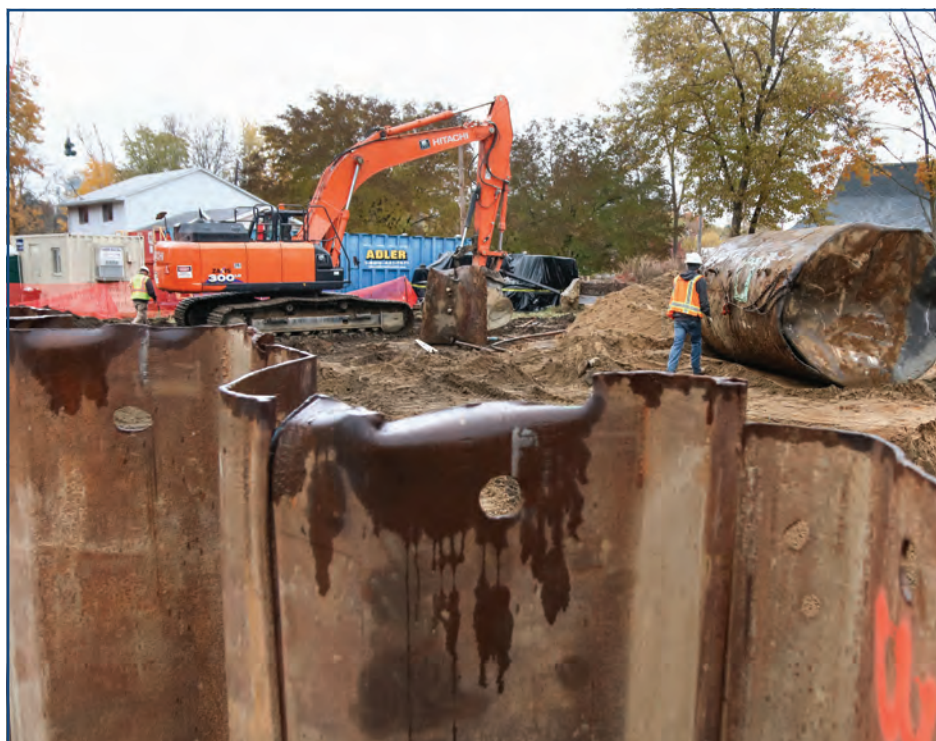
Workers from Environmental Consulting and Technology, Inc. do cleanup work at the old Marathon gas station Thursday, Nov. 1. Here, they take out an underground storage tank. Photo: Hannah Ball
