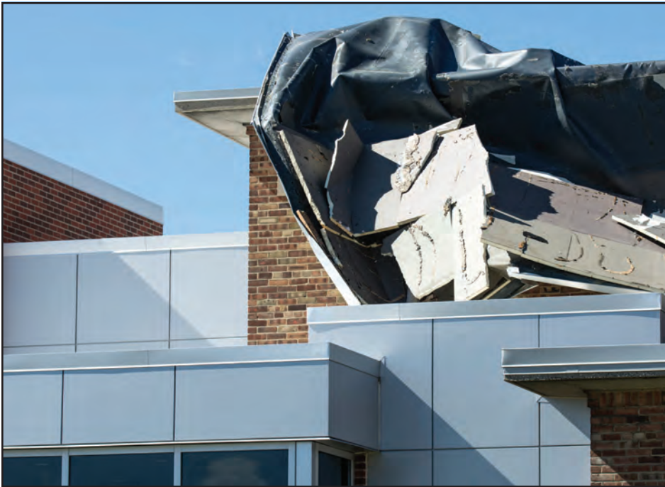
TRI-COUNTY TIMES | TIM JAGIELO Fenton firefighter Frank Carpenter, along with the Fenton DPW carries large pieces of roofing foam away from the scene on Wednesday. Wind gusts up to 60 mph tore the rubber roof membrane from the Fenton Community & Cultural Center on Wednesday.
