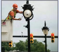
TRI-COUNTY TIMES | TIM JAGIELO Dan Wayne with the Fenton DPW replaces an old bulb in a fixture on Silver Lake Road because the fixture or the pole aren't working properly.
